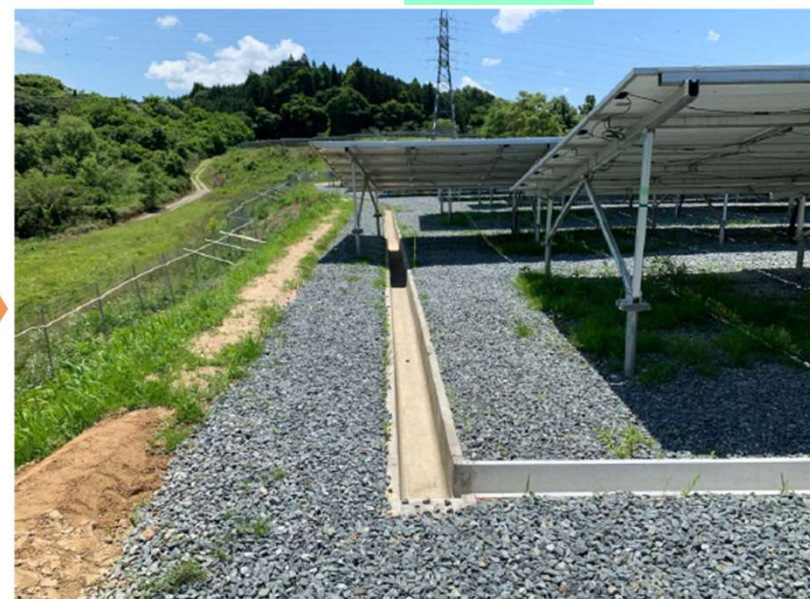
②既設南北U字溝改修 After
