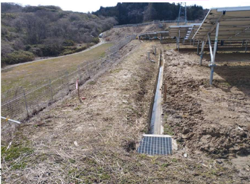
②既設南北U字溝改修工事 Before
